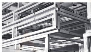
Hot galvanizing structure
